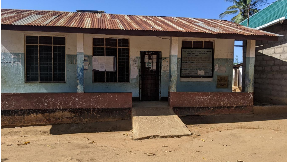
Figure 4-16: Health center in Mpojoni Street with no access to water.
